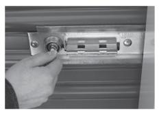
**STEP 1:** Insert the key into the lock with the key horizontal in your hand and the raised tab on the tip of the key in the 3 o'clock position.
