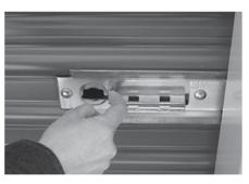
**STEP 4:** With the lock cylinder removed, move the latch to the left to unlatch the door and to the right to relatch it.
